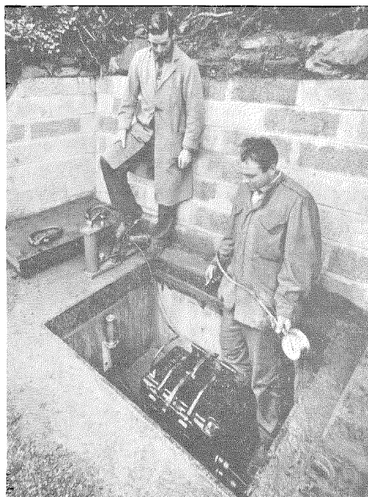
Figure 3—Repeater installed in an early type of housing.
