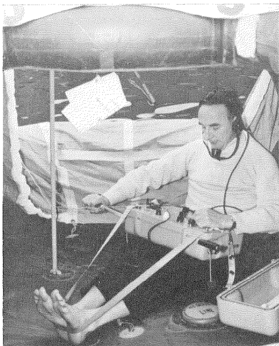
Figure 4—Operation of lifeboat rescue radio set.
