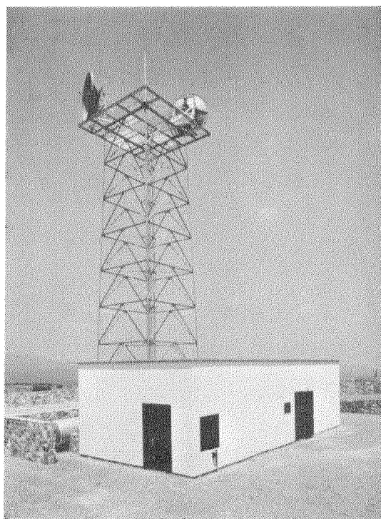
Figure 2—Standard unattended repeater station.
