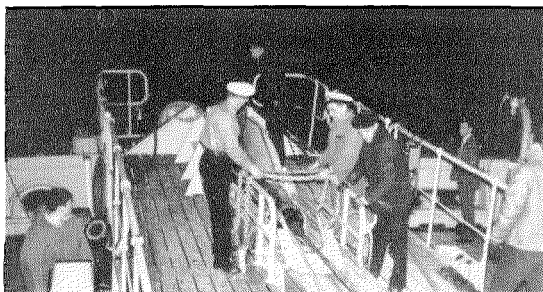
Figure 8—A repeater about to be laid.
