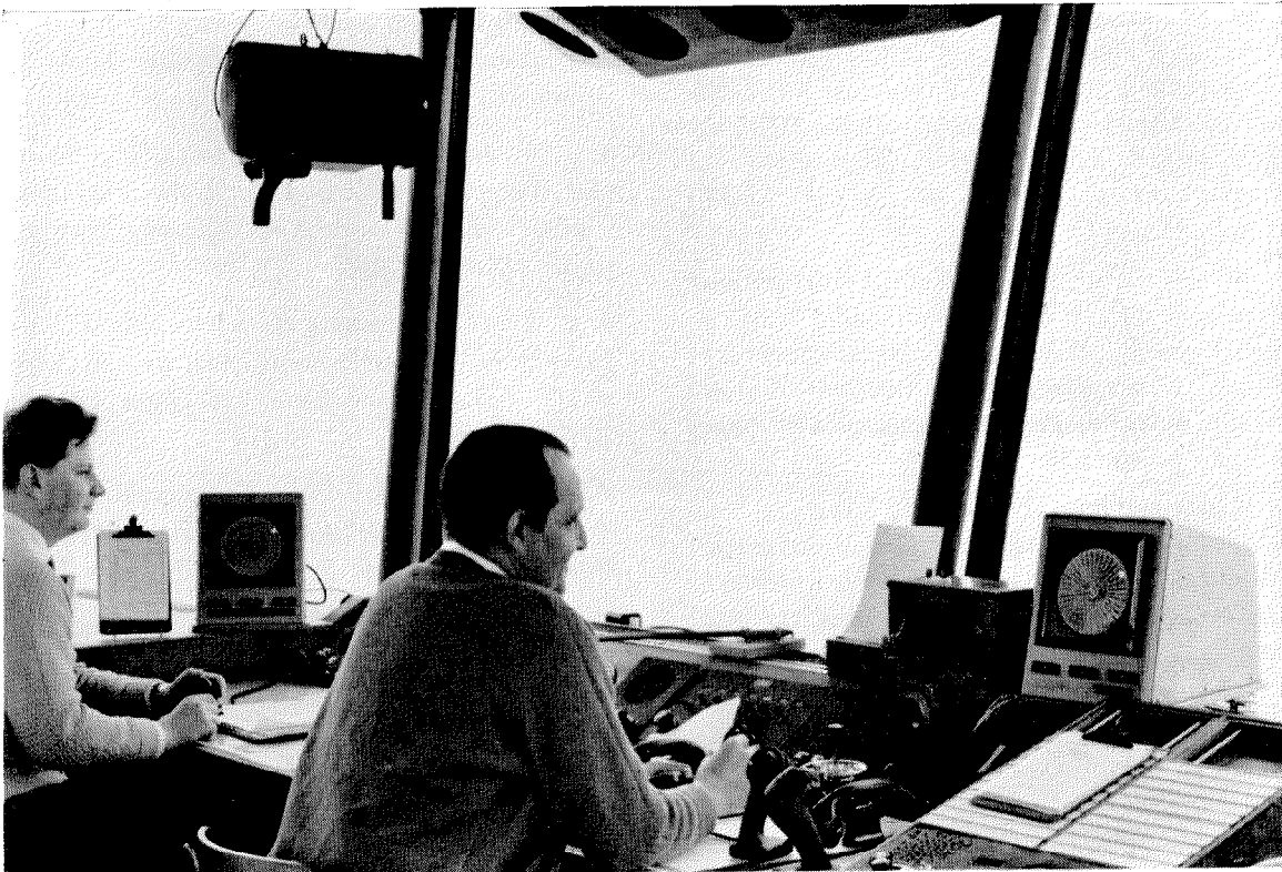
Figure 16—Installation of two slave light indicators in the control tower at an airport.
