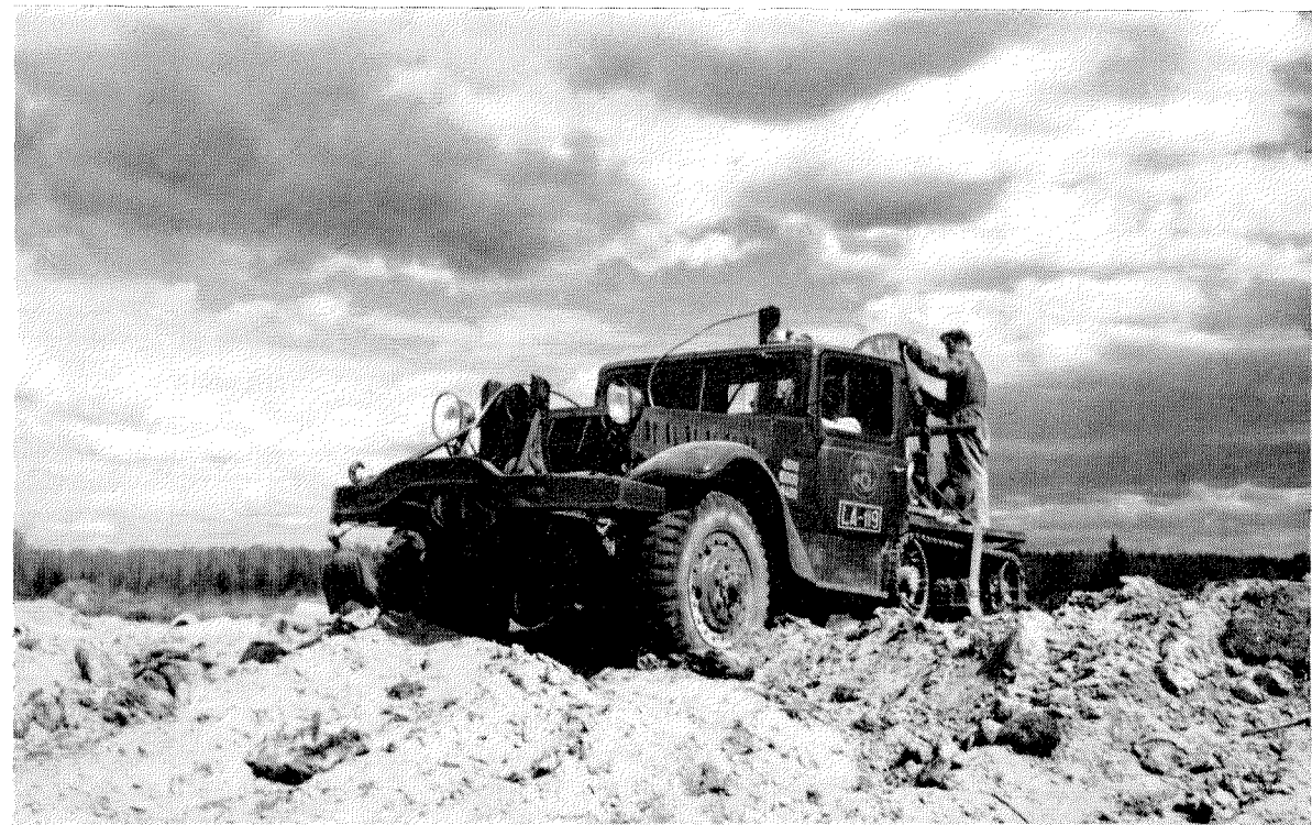
Figure 6—Half-track vehicle used for laying cable in trench.
