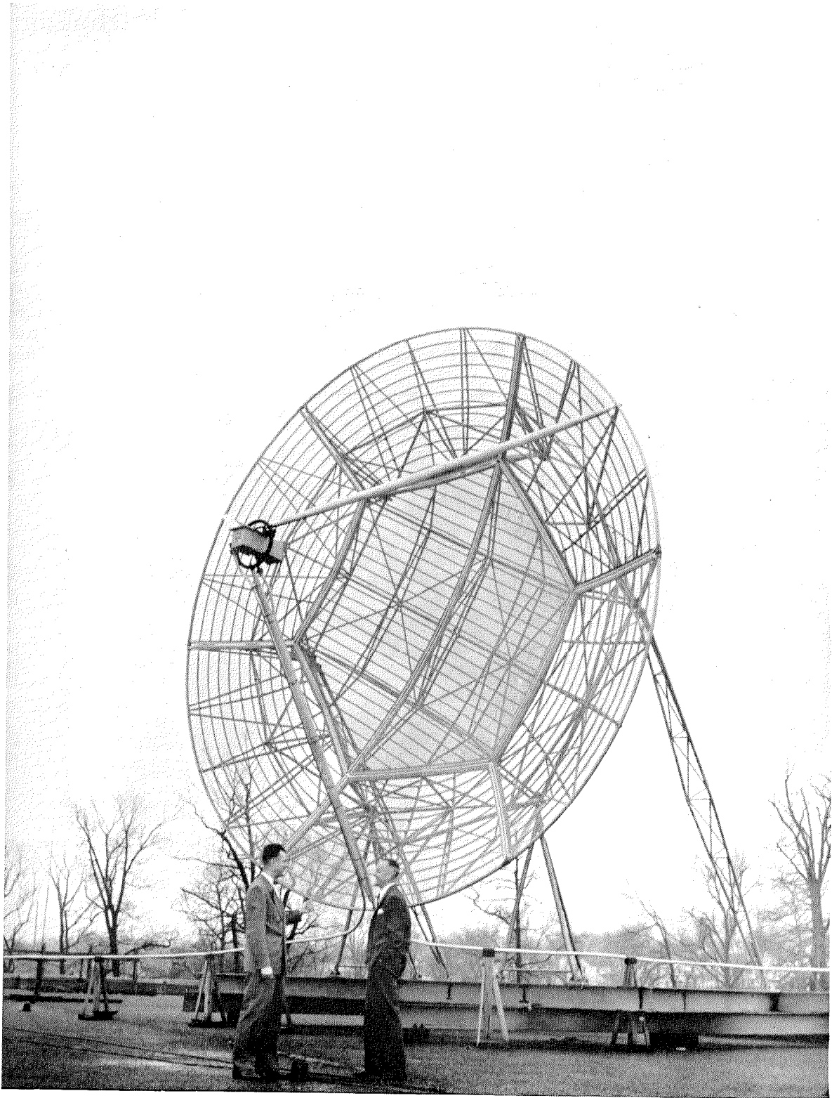
Figure 3—View of 28-foot (8.5-meter) paraboloidal antenna with dual polarization horn.
