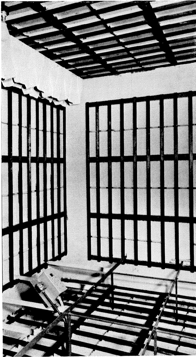
Figure 1—The walls have been covered with Celotex board and a lattice of wooden battens has been erected to support the fibreglass wedges that provide most of the sound absorption.
