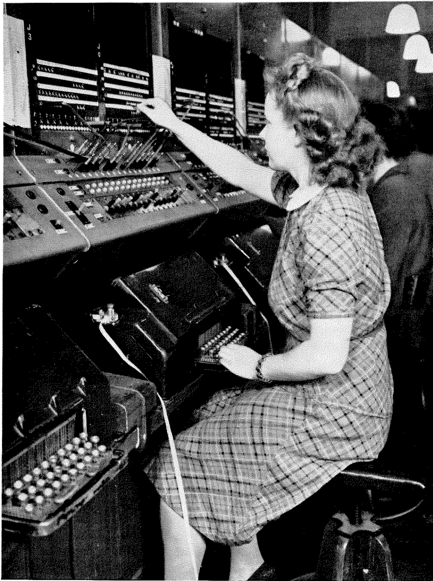
Manual teleprinter switchroom at Manchester, England.
