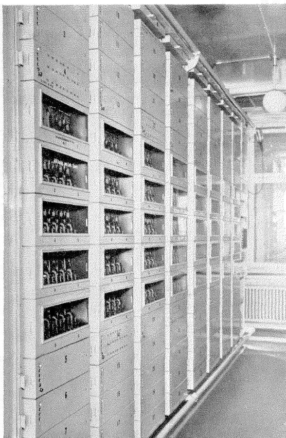
Fig. 5—Selective trunk circuits from 7-A1 local exchanges.
