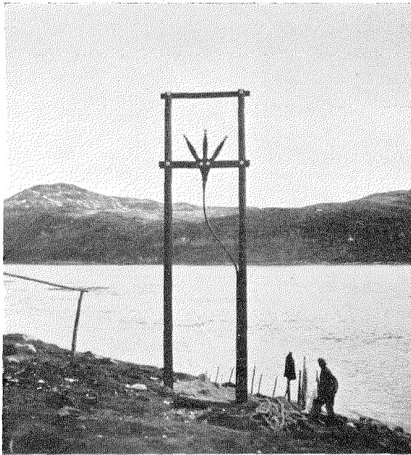
Cable installation at 71 degrees north latitude. The pot-head termination of the 3-phase cable is supported on the lower wooden cross arm.
