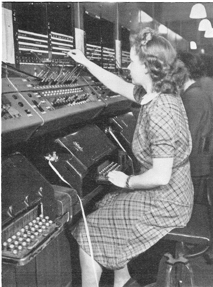
Teleprinter switch-room in Manchester.
