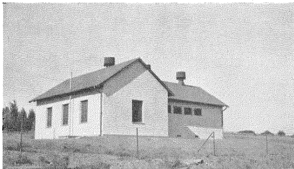
Fig. 13—Typical repeater station building.
