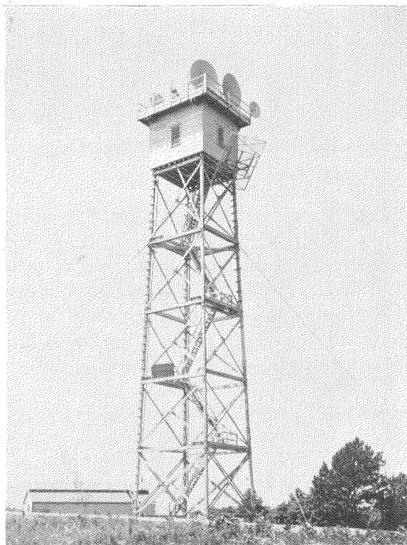
Fig. 16—100-foot wooden tower at Telegraph Hill, New Jersey.
