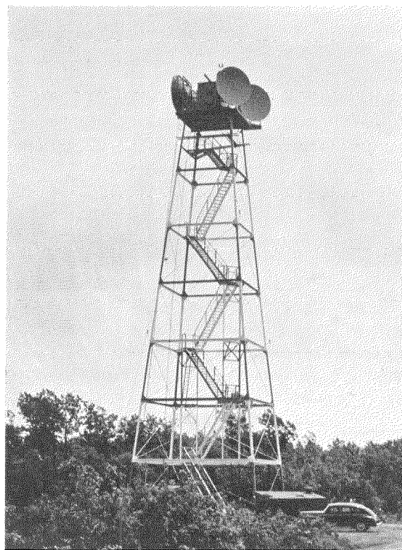
Fig. 18—100-foot steel tower at Laurel Hill, New Jersey.
