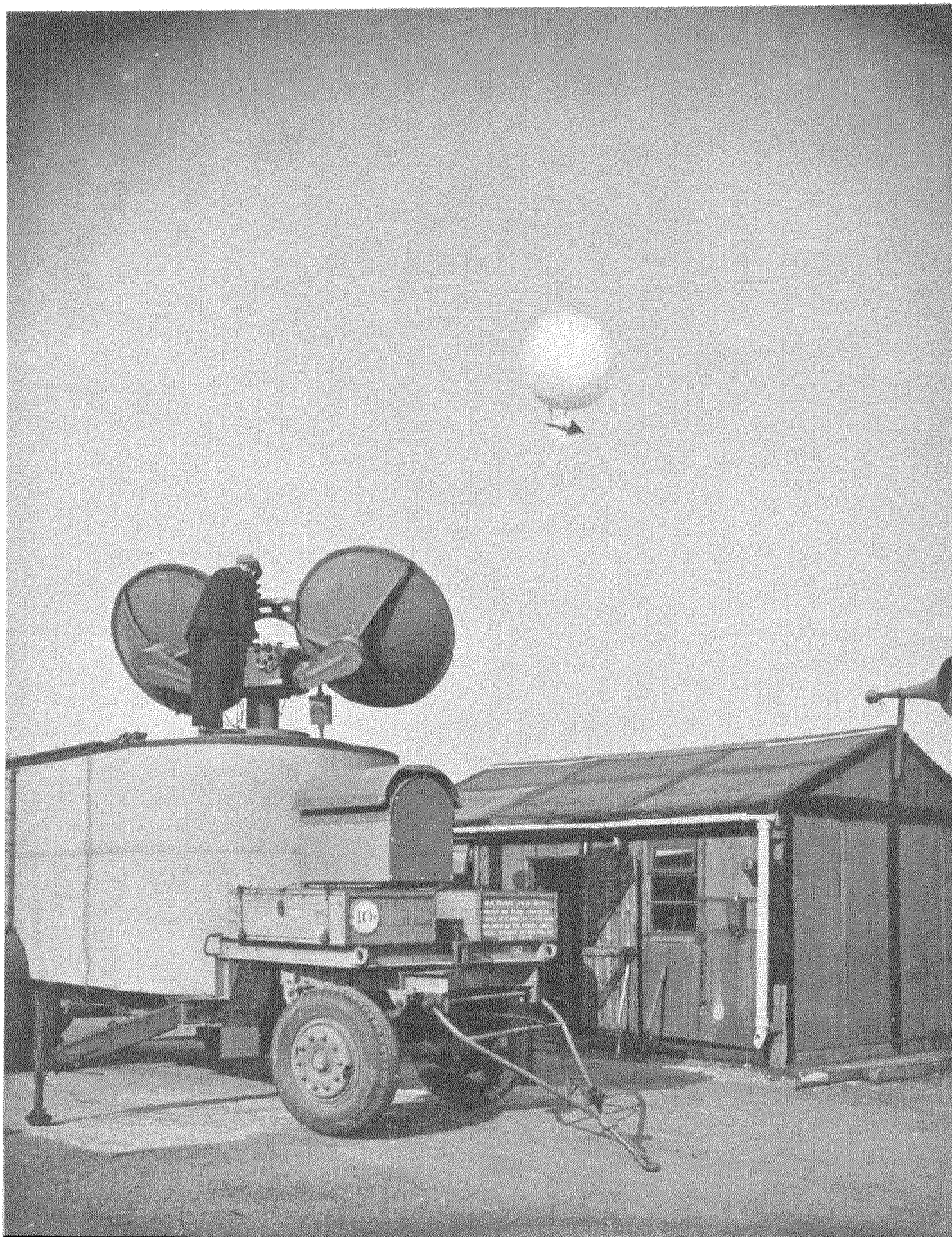
METAL-TAILED BALLOON USED IN TESTING STANDARD TELEPHONES AND CABLES, LTD. (LONDON) EQUIPMENTS FOR THE ACCURATE DIRECTION OF ANTI-AIRCRAFT GUNFIRE.
