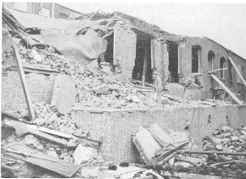
North Woolwich factory after a flying-bomb incident in 1944. The man is standing on a surface shelter which was undamaged except for the blocking of escape exits by debris.
