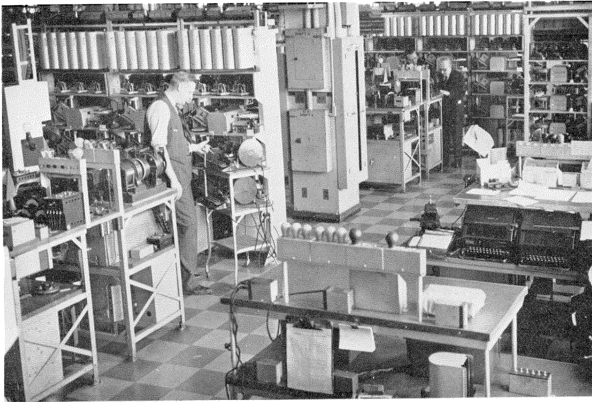
Fig. 2—Varioplex Central Office equipment.
