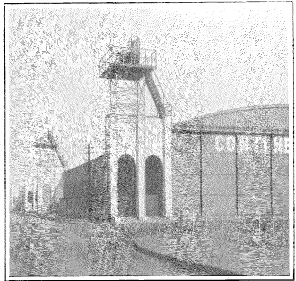
Fig. 4—View of the reflector towers at Lympe, England, terminus of the Anglo-French micro-ray link between Lympe and St. Inglevert, France. It represents the first commercial micro-ray installation, designed to operate on a 17-centimeter wavelength with sharply concentrated beams.
