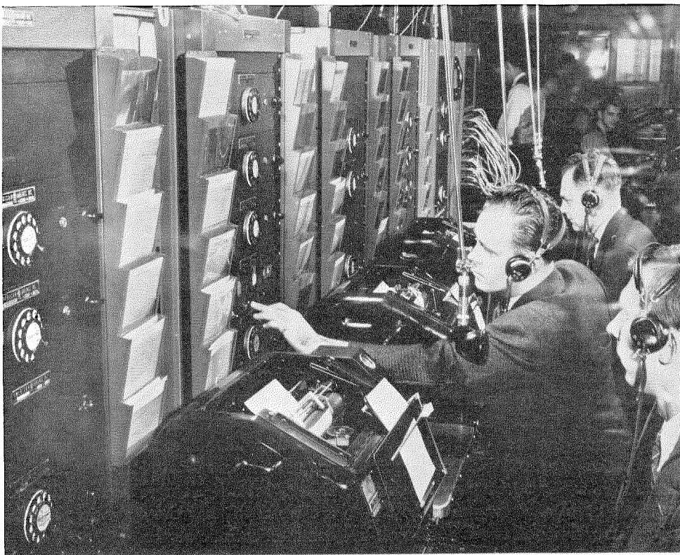
Fig. 3—Radiotelephone Operating Positions, Communications Center of American Airlines, La Guardia Field, North Beach Airport, New York.
