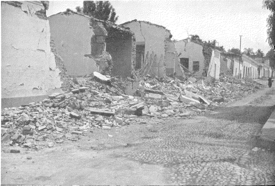
A Street in Colima After Partial Clearance.
