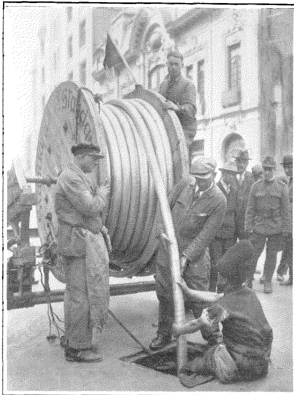
Feeding 2424 Pair Cable into manhole, Bucharest, Rumania. This cable, containing the largest number of pairs ever manufactured commercially for a customer in any country in the world (1932), was supplied by Standard Telephones and Cables, Ltd., London.
