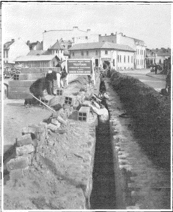
Placing Clay Conduit in Bucharest.
