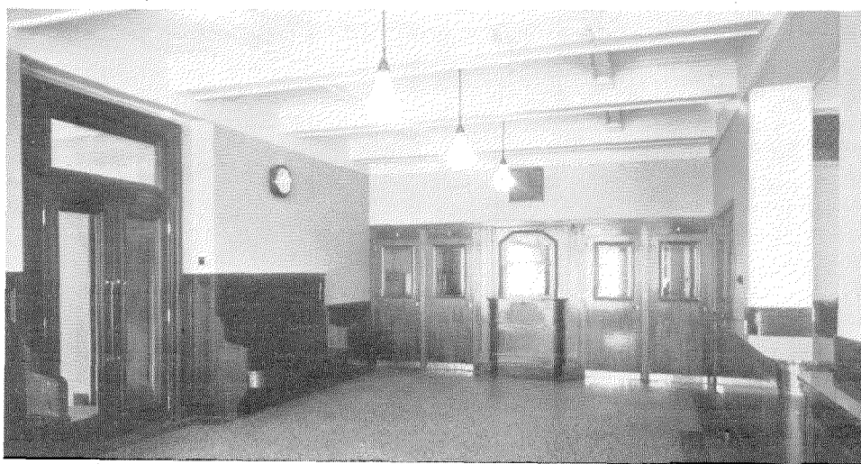
Cluj Commercial Office with Pay Stations in Rear.
