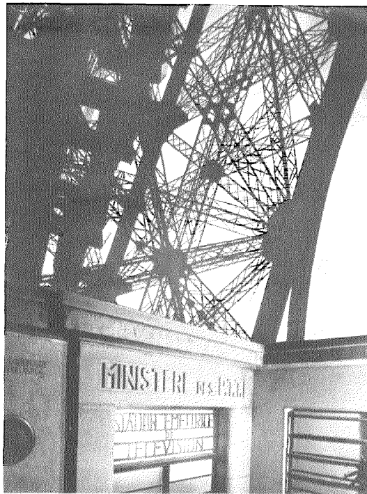
Fig. 3—Main Entrance to the Eiffel Tower Television Transmitter.
