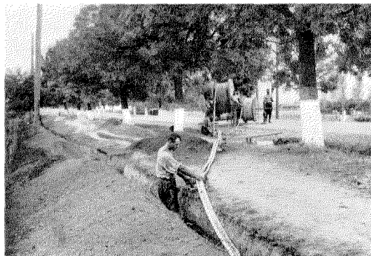
Pulling-in the Two Armoured Cables.
