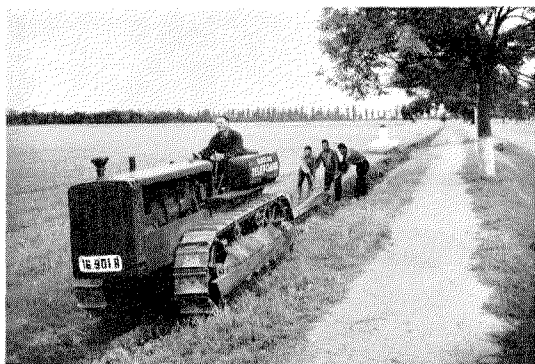
Trenching with Tractor-drawn Plough.
