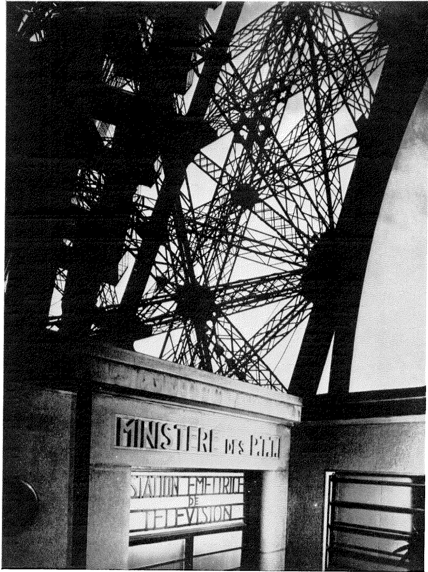
Entrance to the French P.T.T. 30 kW Eiffel Tower Television Station.
