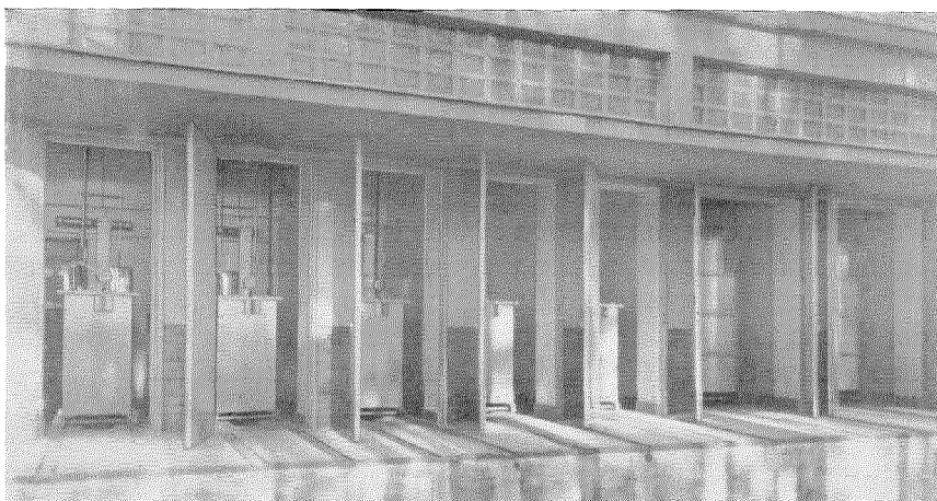
Fig. 18—Final high frequency amplifier plate feed reactors.
