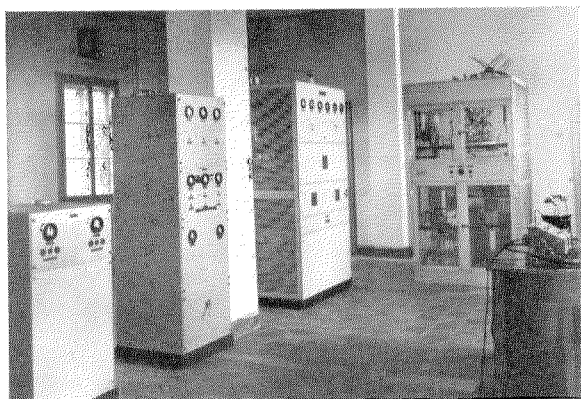
Fig. 4—Transmitter Room at Varna. From left to right : Low Voltage Rectifier, Oscillator-Modulator Unit, Power Amplifier and High Voltage Rectifier.
