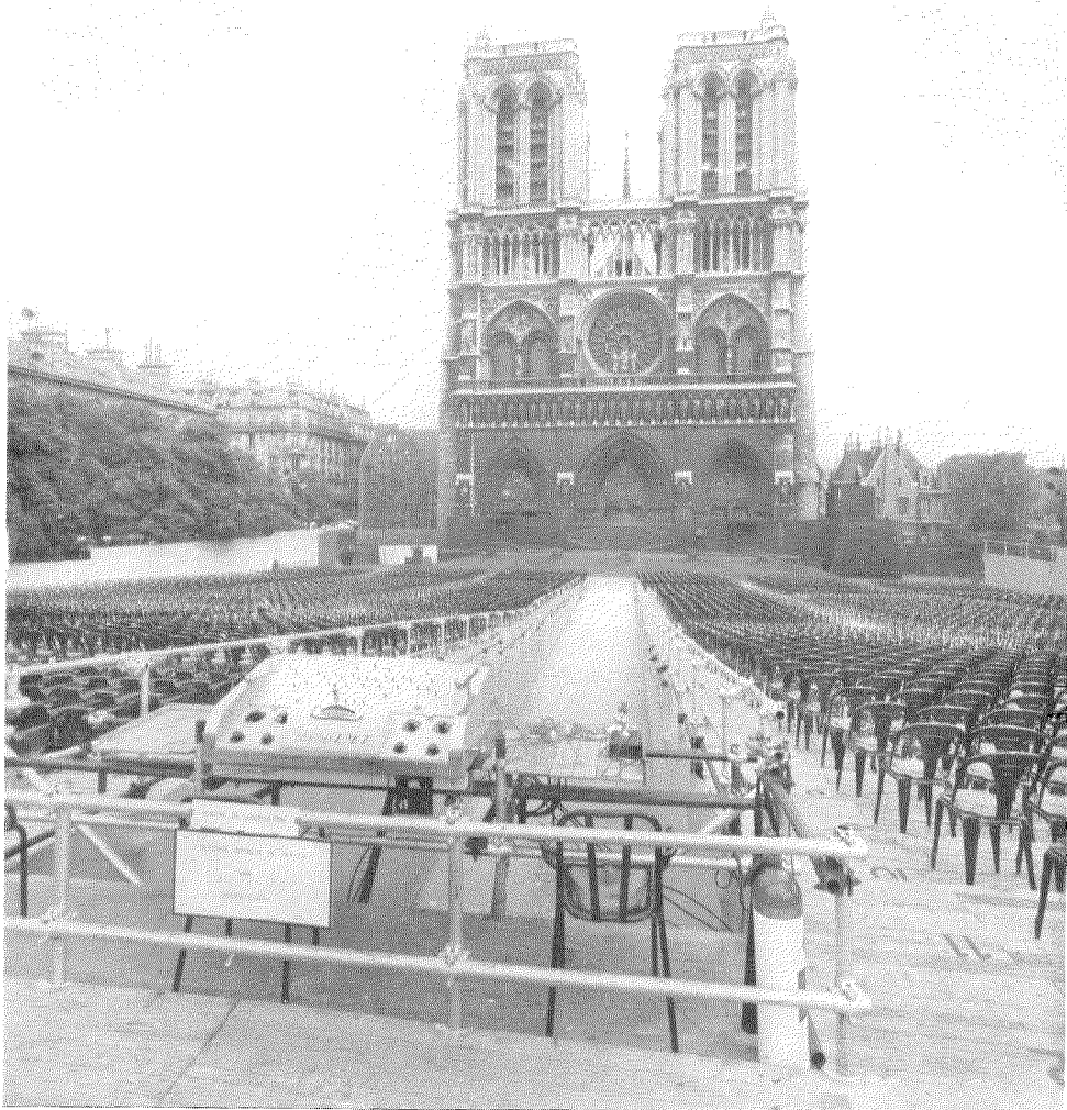
Notre Dame Cathedral showing the Stage and about One-Half of the Auditorium. The Operating Switchboard is in the foreground and the Auditorium Loudspeakers are Visible at the Extreme Left.
