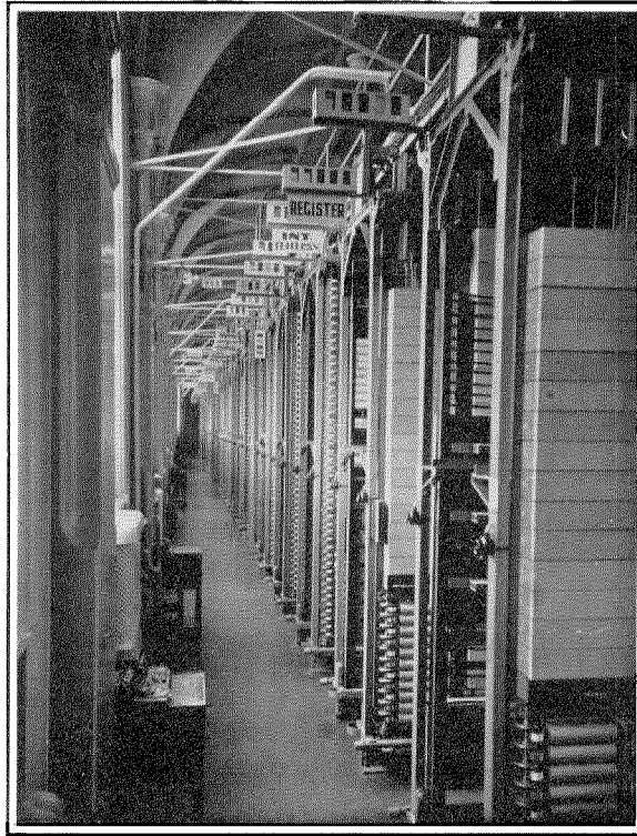
Figure 6—Teréz Automatic Exchange—Machine Switching Room, Lower Level.
