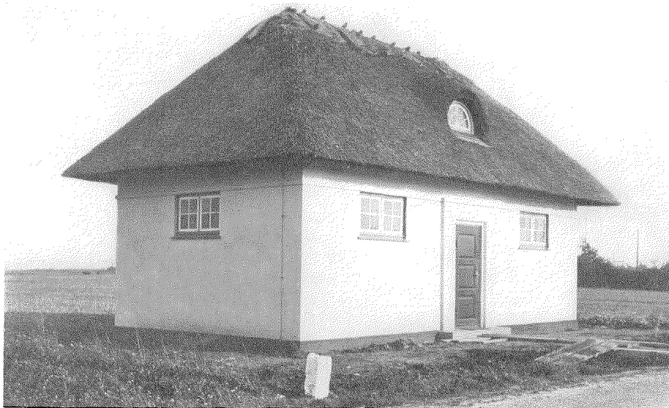
Fig. 13—Brondby Vester District Exchange—Denmark—600 Lines Capacity.
