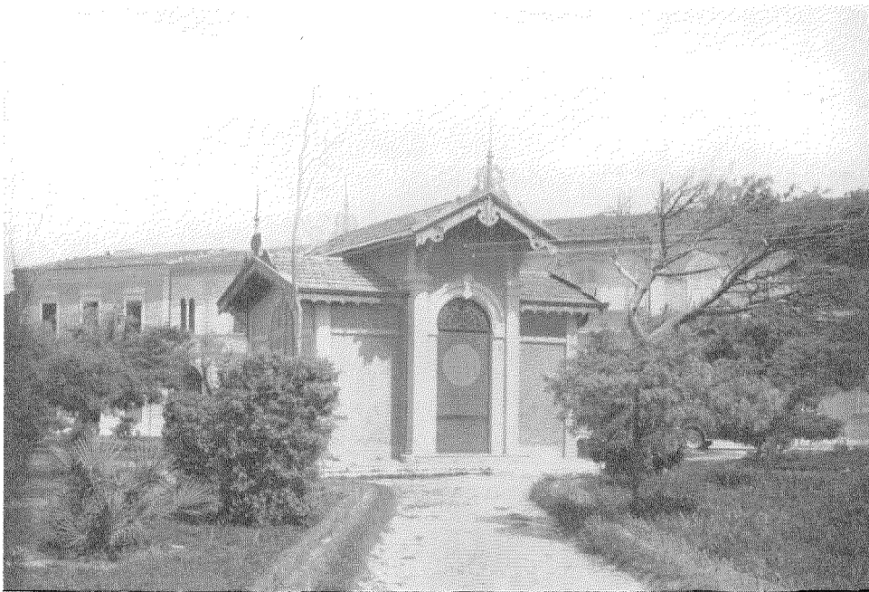
Fig. 10—Marina di Pisa District Exchange—Pisa Rural Area—Italy—500 Lines Capacity.
