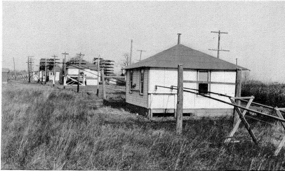
Figure 4—Phoenixville Installation Showing Conductors Entering Test House.
