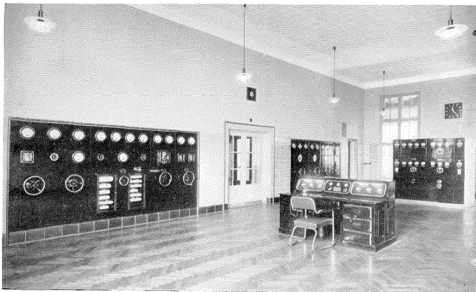
Figure 3—(Upper) Oscillator-Modulator Unit, Control Desk and Front of High Voltage Radio Frequency Cubicle. (Lower) Power Board and Water Control Board.
