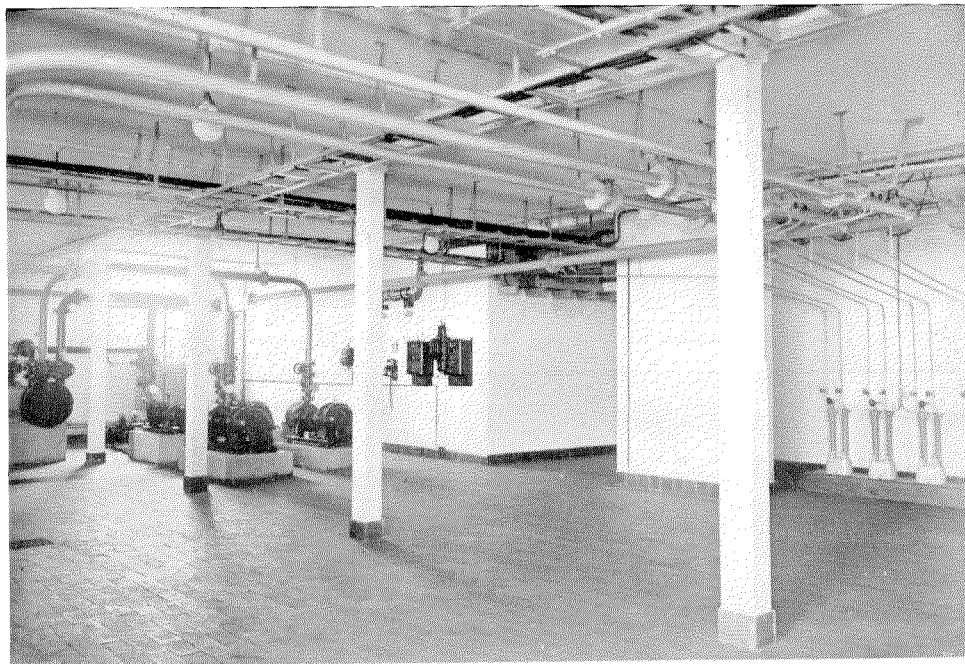
Figure 4—The Basement at Kalundborg.
