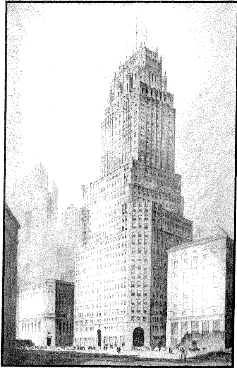
INTERNATIONAL TELEPHONE BUILDING 67 Broad Street, New York
