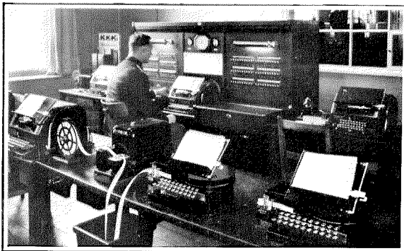
Figure 5—Automatic Transmitting Device at Berlin Police Headquarters
