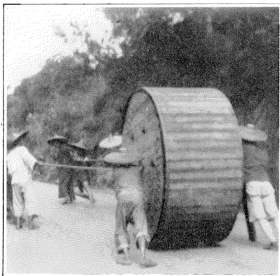
Figure 8—Distributing Drums Along Road in British Territory.
