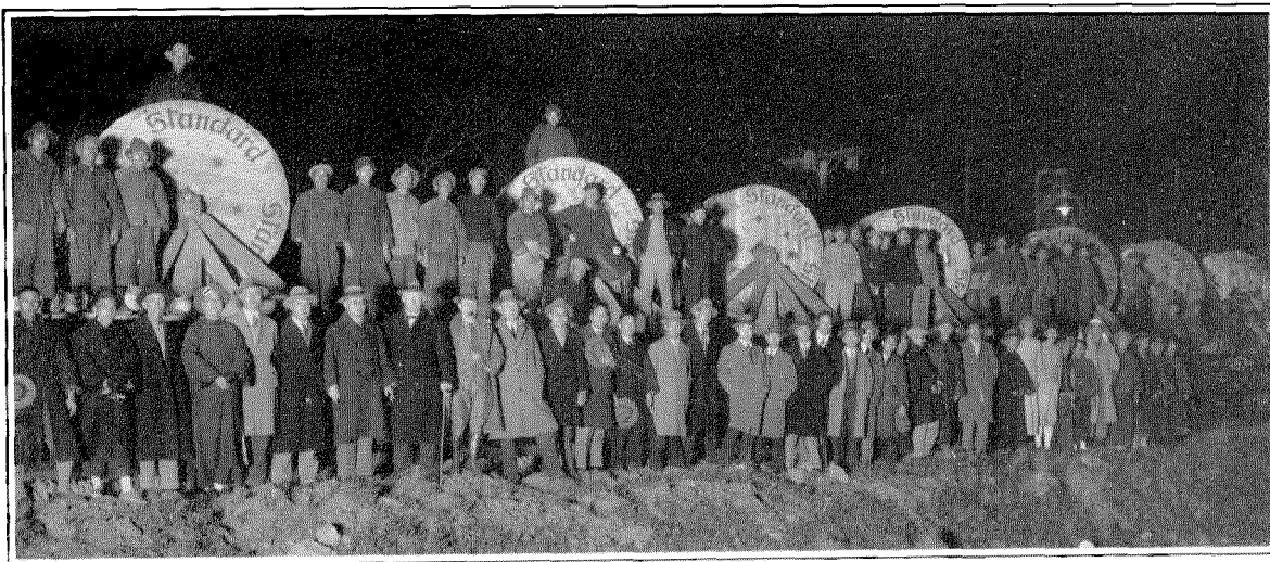
Figure 10-b—Cable-laying Train. First Night Out Just Before Starting Laying.
