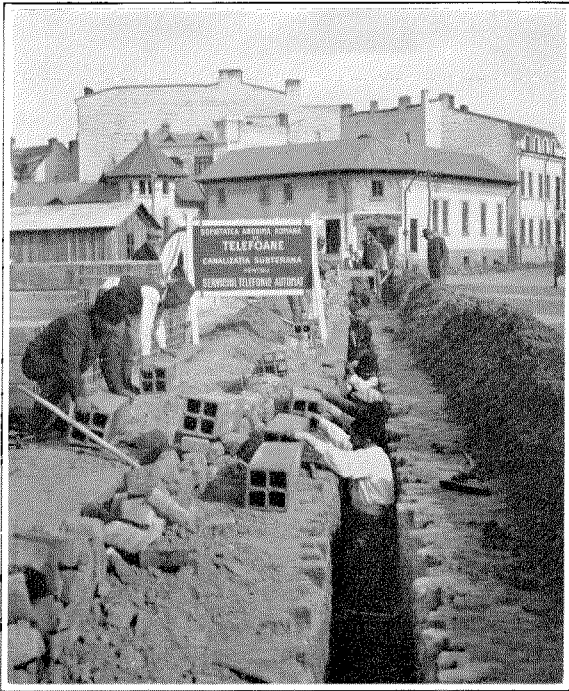
Underground Conduit Work in Progress in Bucharest.
