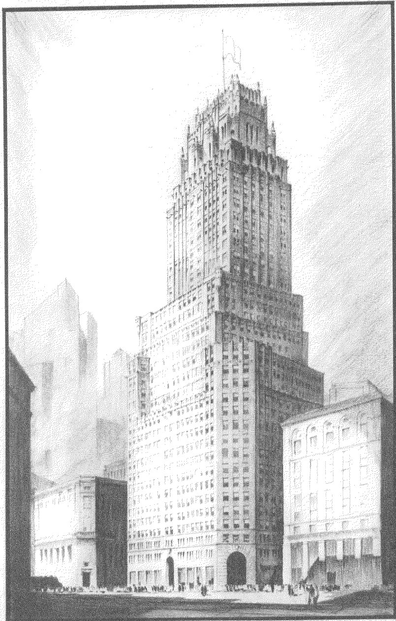
INTERNATIONAL TELEPHONE BUILDING 67 Broad Street, New York
