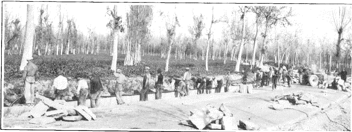
Figure 1—Cable-laying Near Naples.
