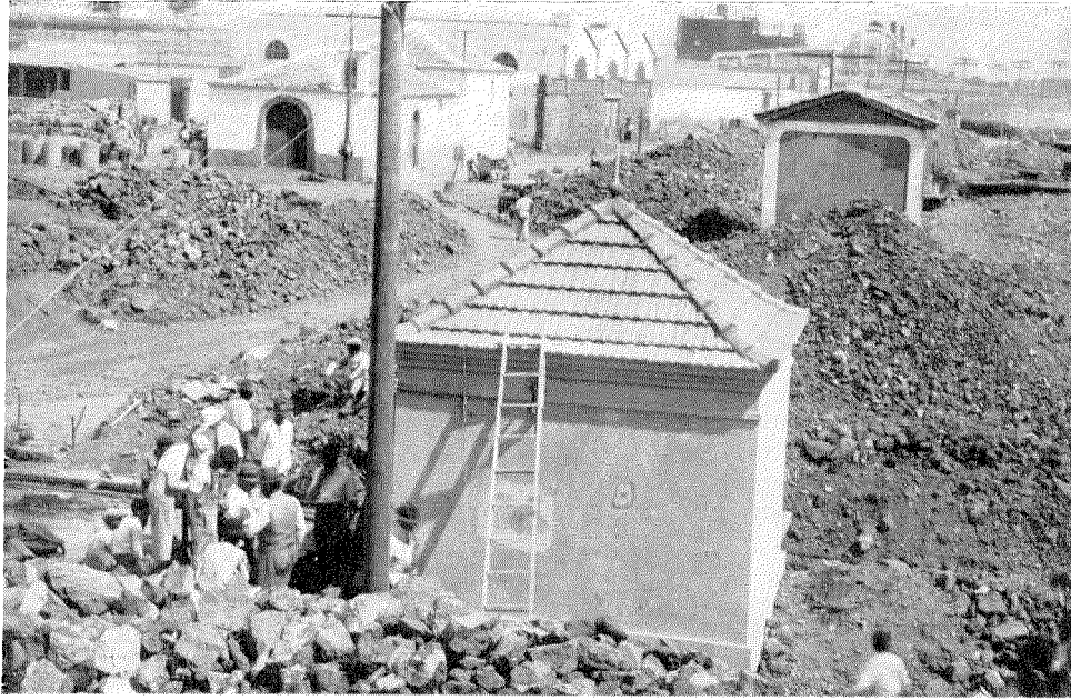
Figure 5—Cable Hut, Santa Cruz, Tenerife.
