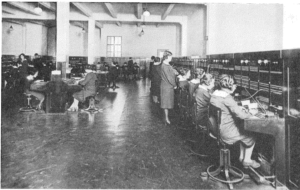
Figure 11—New Toll Switchboards, Barcelona.
