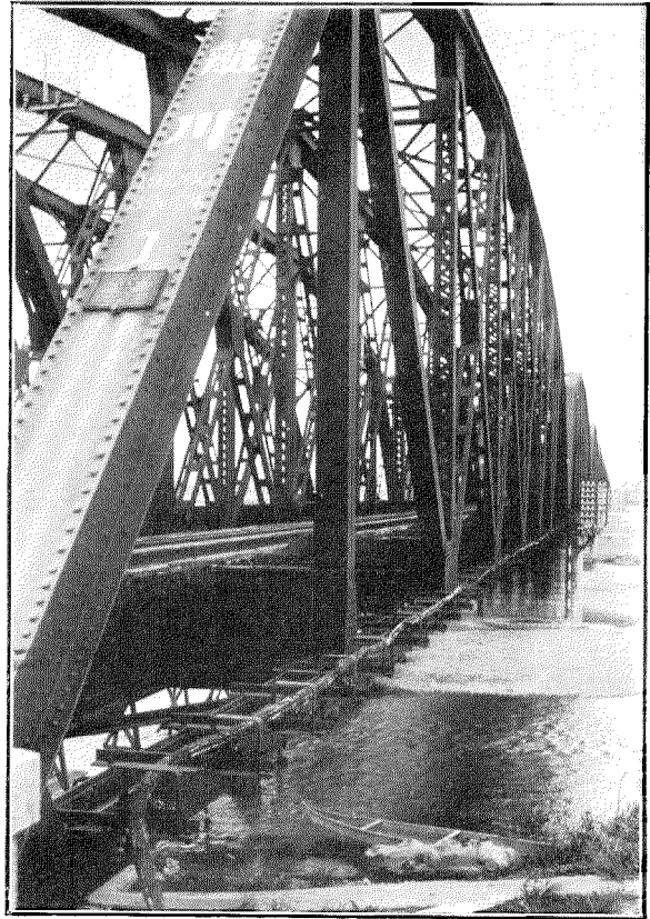
Figure 11—Armoured Cable Placed on Railroad Bridge Across the Tenryu River.
