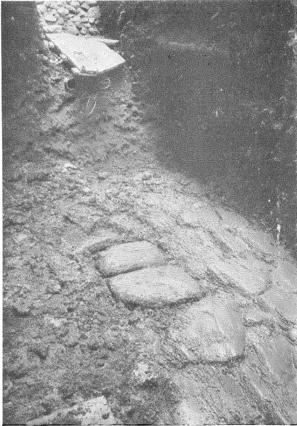
Traces of the Old Roman Road Found at a Depth of 3 Meters from the Level of the Actual Street while Digging a Manhole.
