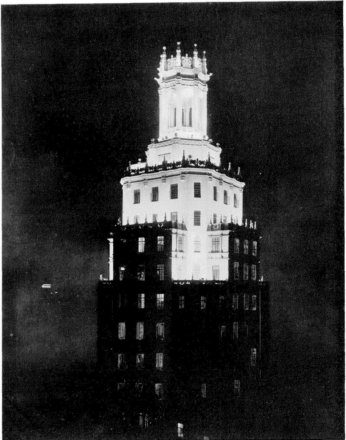
New Building of the Cuban Telephone Company, Havana. It is the highest building in Cuba, consisting of ten stories and a three-story tower. The illustration shows the results of the recent installation of floodlighting equipment.
