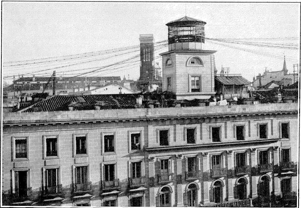
Figure 1—Overhead Wires and Cables Entering the Mayor Manual Exchange, Madrid, through a Tower on the Roof. The housetop construction, typical of the old outside distributing plant, may be seen on the horizon.
