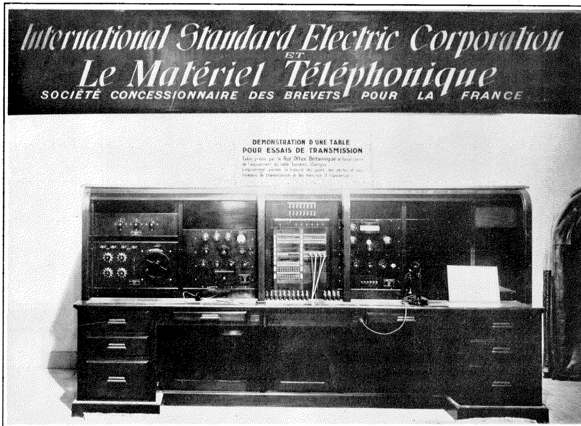
Figure 17—Repeater Station Test Desk
