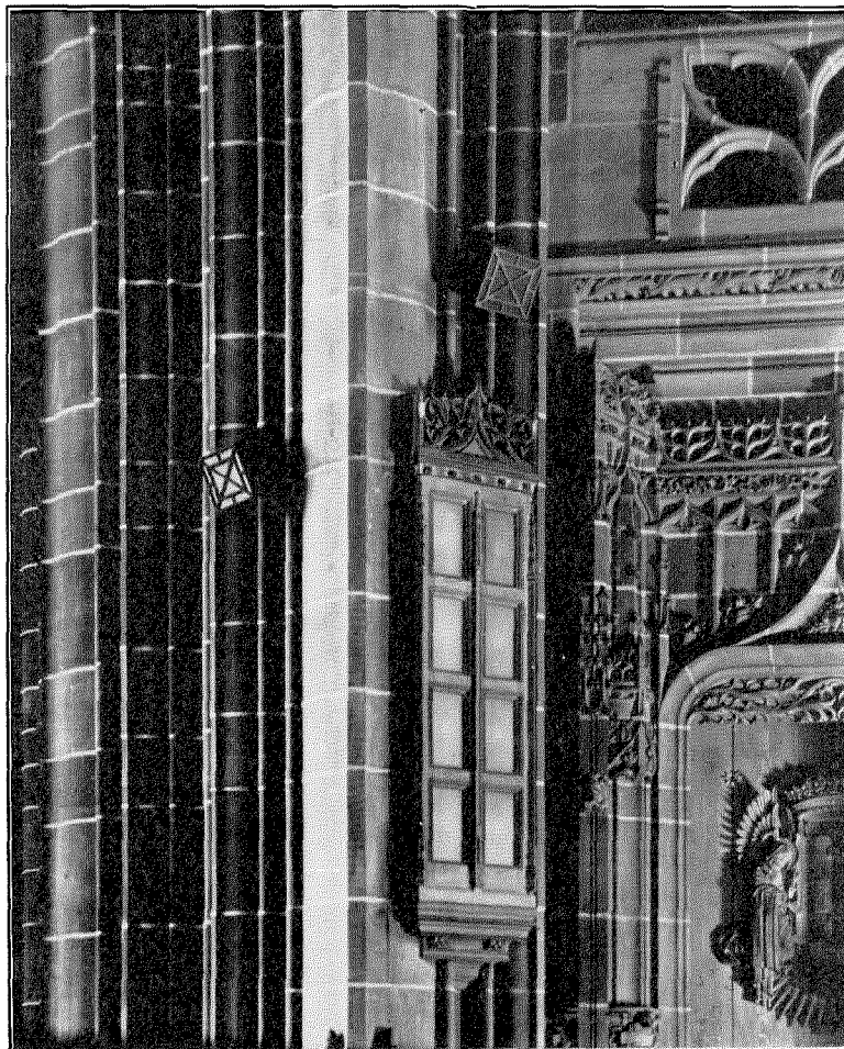
Figure 3—Column on North Side of Chancel, Showing Voice-projectors in Position
