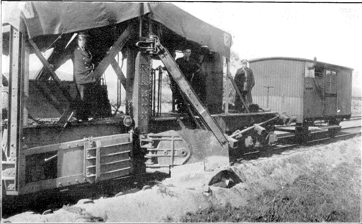
Figure 4—Trenching Machine at Work
