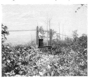
Fig. 8—Toll cable line showing loading coil case
