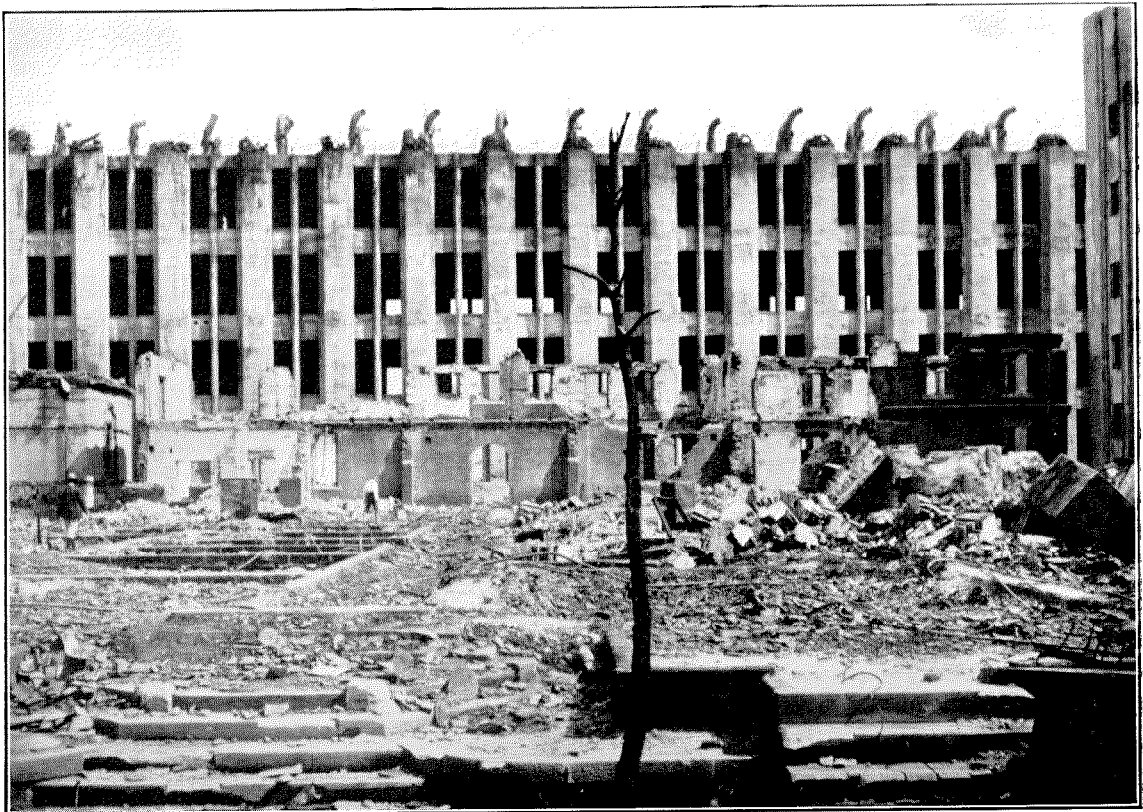
Figure 20—New Tokio Central Telegraph Office After Fire. In Course of Construction
