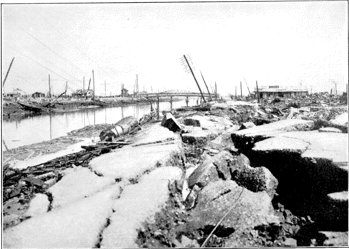
Figure 1—Cracks in Ground Near a River in Yokohama—Telephone Pole Near Center of Picture
