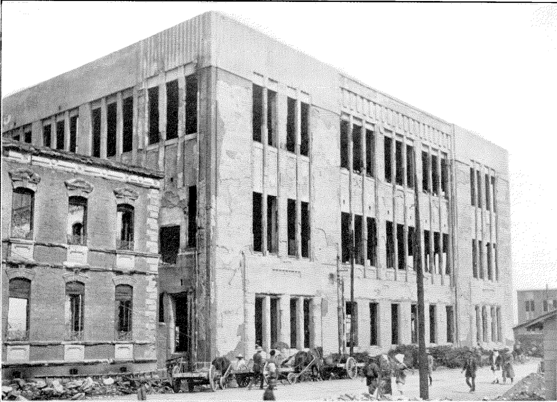
Figure 8—Outside View of Building After Fire, in which were located two units of Telephone Central, Hamacho and Horidome, Tokio. Reinforced concrete building to be used again as Common Battery Office. Brick building to left is Central Naniwa
