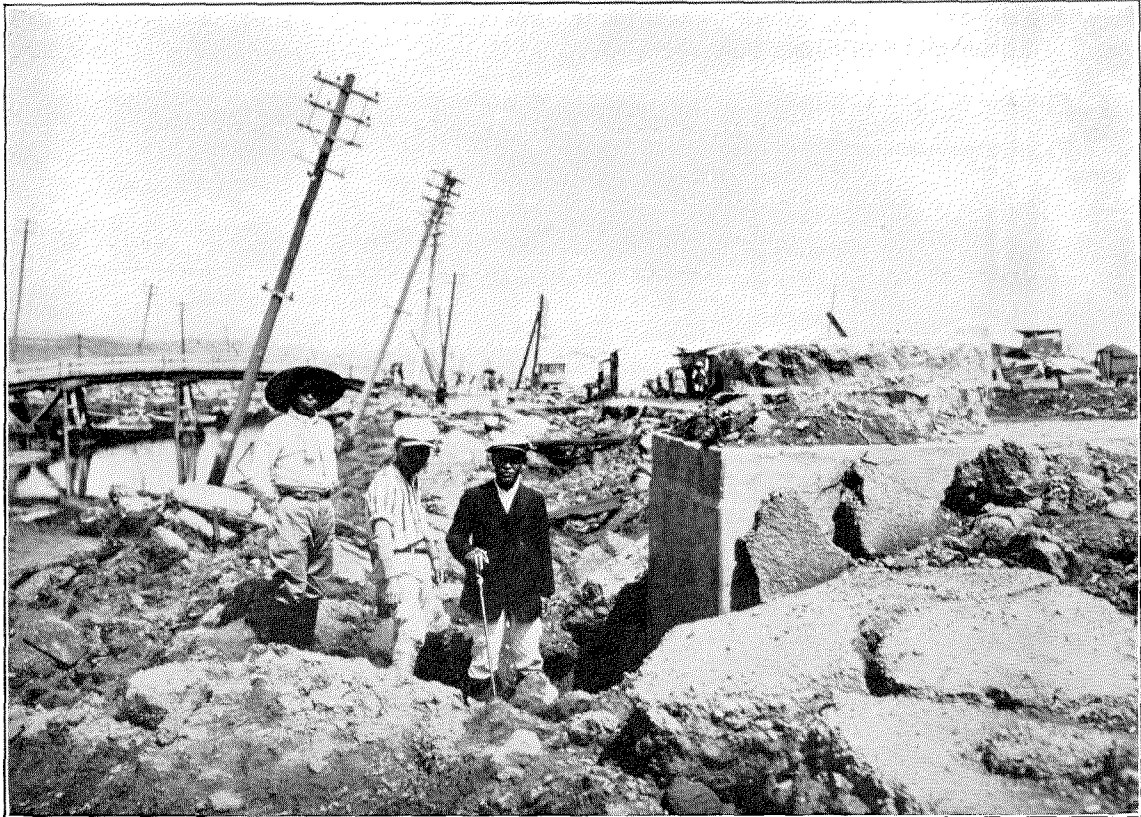
Figure 17—Manhole Near River Bank in Yokohama Remained Unsunken. Head of Manhole Projecting Above Road Surface
