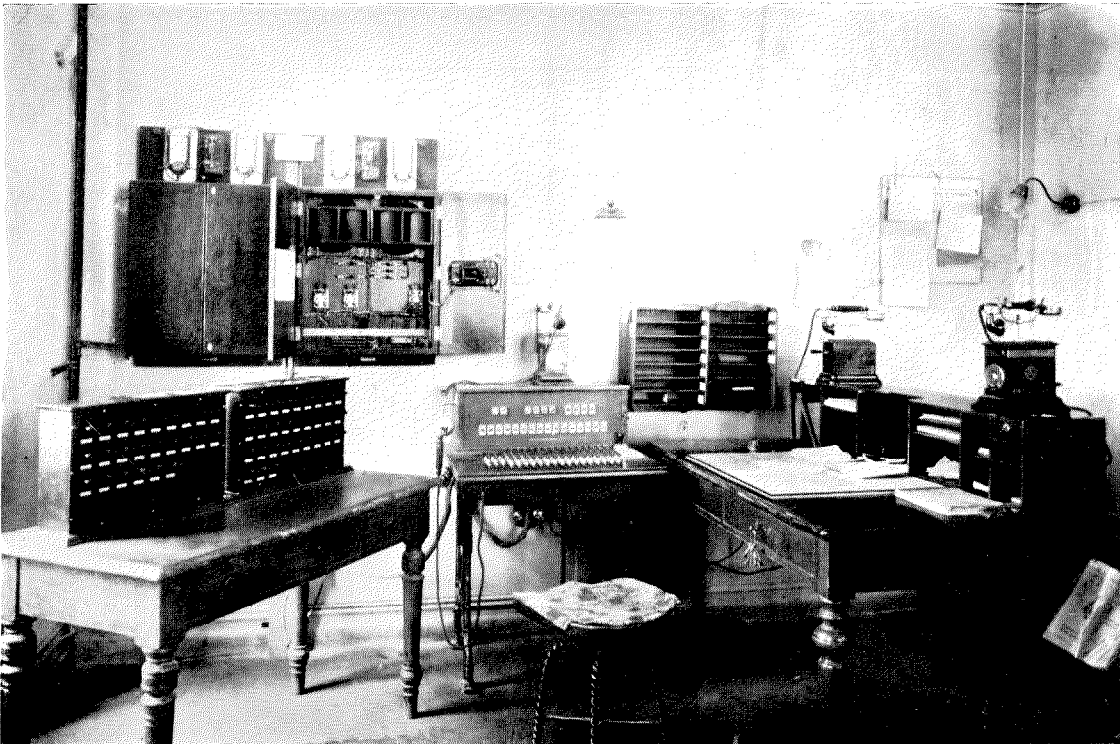
Figure 13—Telephone Train Dispatching—Goteborg Dispatching Office, Sweden
