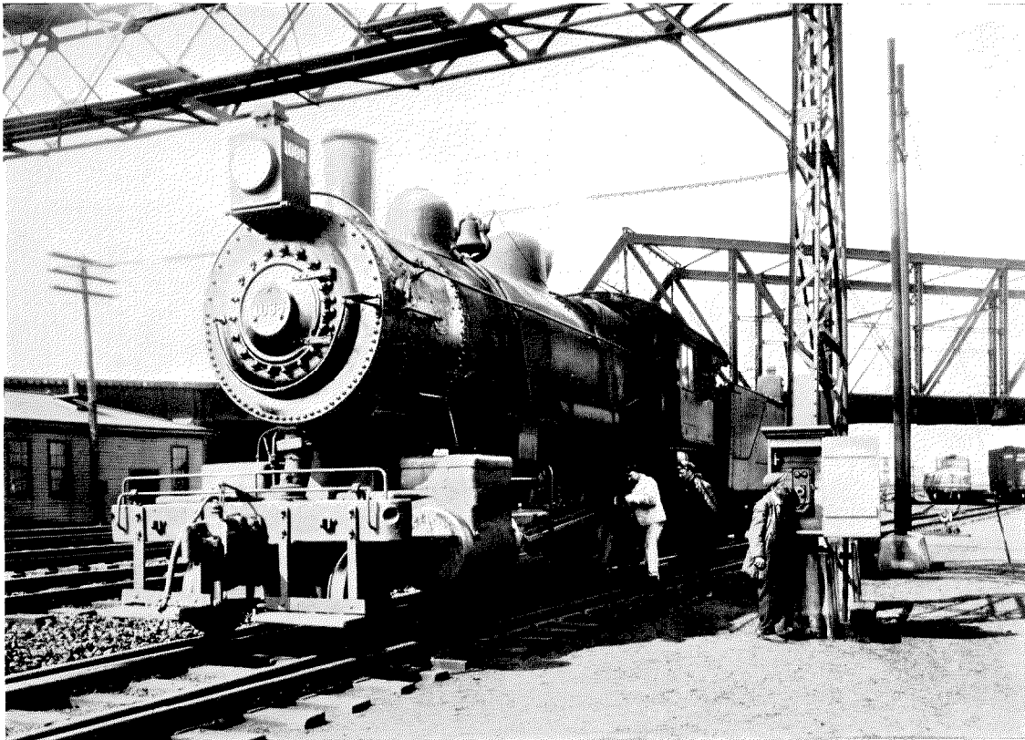
Figure 6—Telephone Train Dispatching—Siding Telephone
