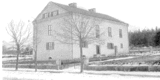
Figure 18—Enköping Repeater Station
