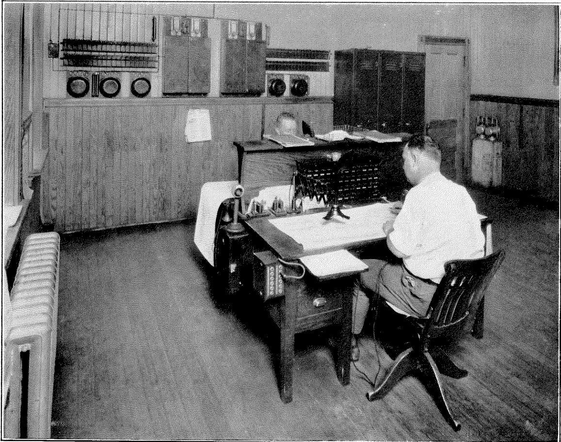
Figure 18—Train Dispatcher's Office. Loud Speaking Equipment Installation
