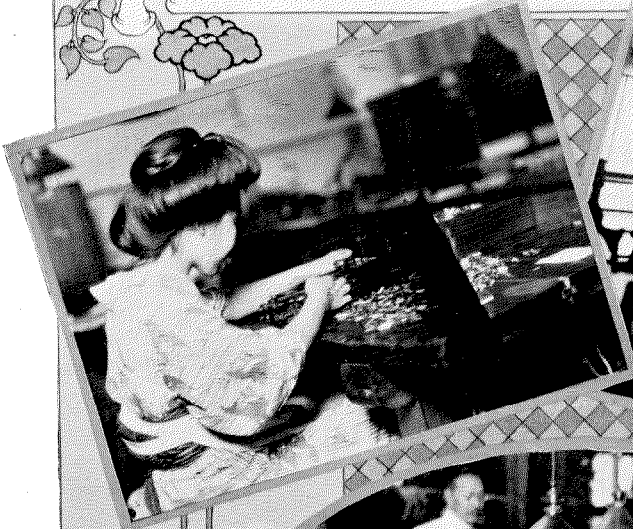
Making the tiny switchboard lamps
