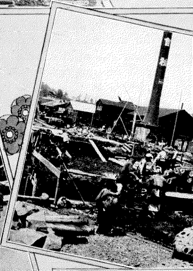
Inside the compound -preparing for new building construction
