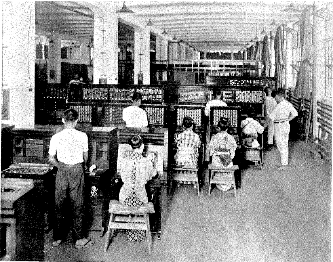
Nippon Electric Company—Switchboard Assembly
