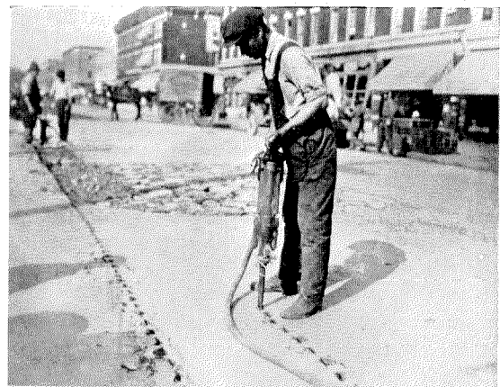
Figure 22—Air Gun Cutting Asphalt
