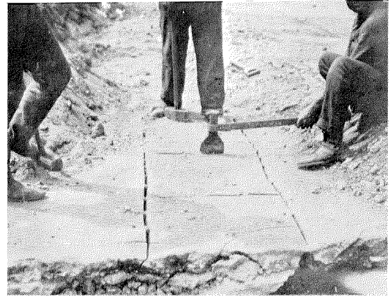
Figure 24—Manual Method of Cutting Asphalt. Contrast with Figure 22
