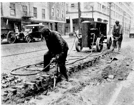
Figure 21—Removing Granite Blocks and Breaking Concrete Base
