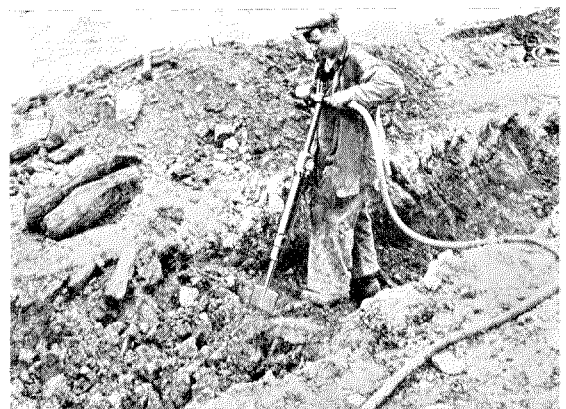
Figure 25—Pneumatic Spade Replacing Hand Pick Method of Loosening Hard Soil
