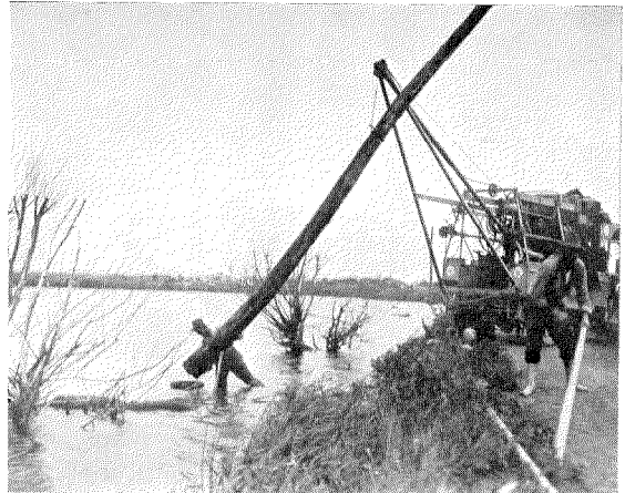
Figure 5—Derrick Operating Under Difficult Conditions
