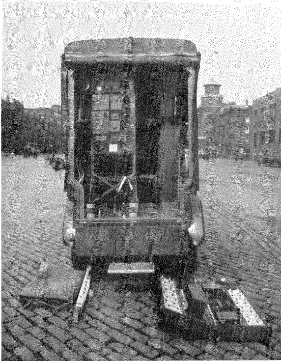
Fig. 5. Mobile Public Address System—Amplifiers and Control Panels
